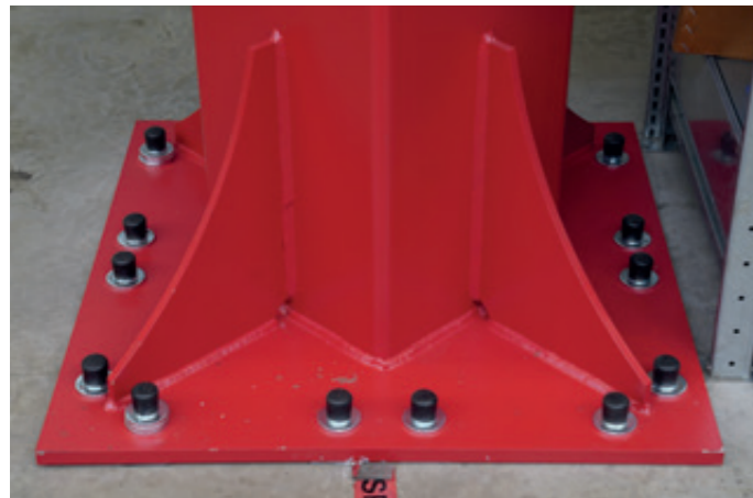
Dynamic dowel fixing Anchored directly to the hall floor via a base plate.
