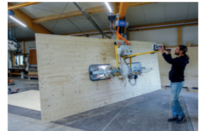
VacuPoro VP-90E-250KG Moving blockboards from an upright shelf system onto a panel saw.
